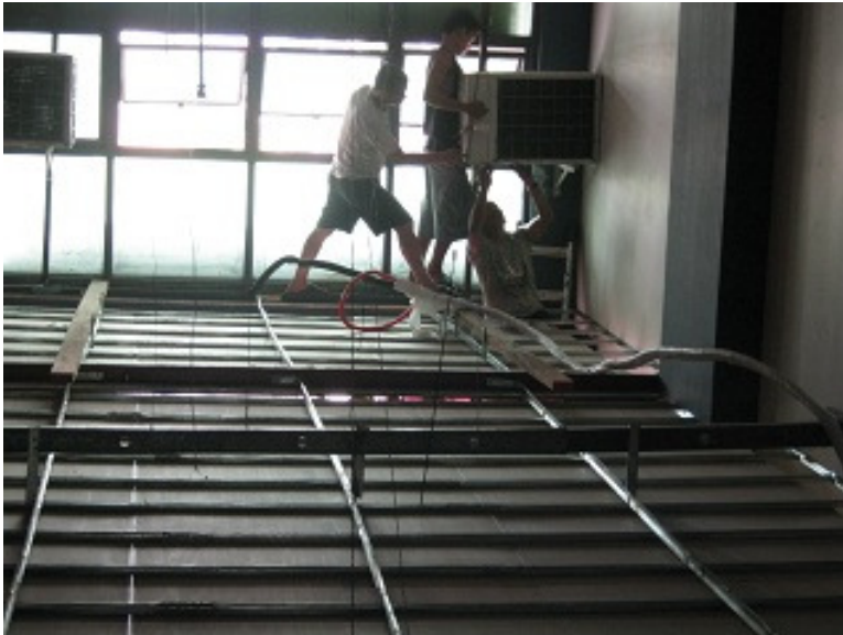
Installation of the air condition compressor
