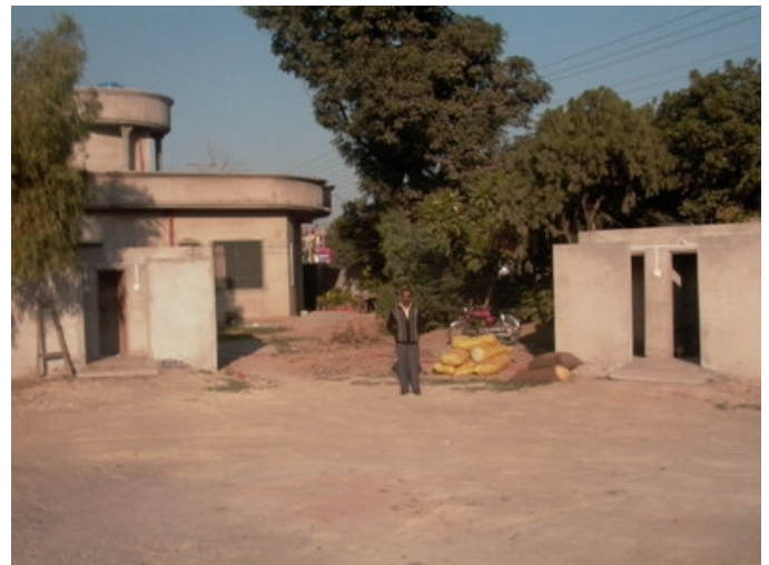
Part of the new area and washrooms
